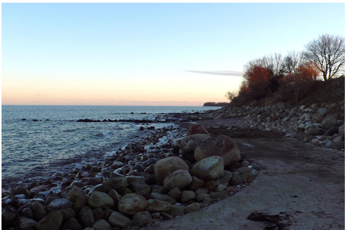
Figure 8.26 At Klausdorf Strand Camping Site. Upper left: headland protected by revetment. Upper right: boat ramp between two groynes. Lower: revetment and groynes towards SSE, shingle/boulder beach
