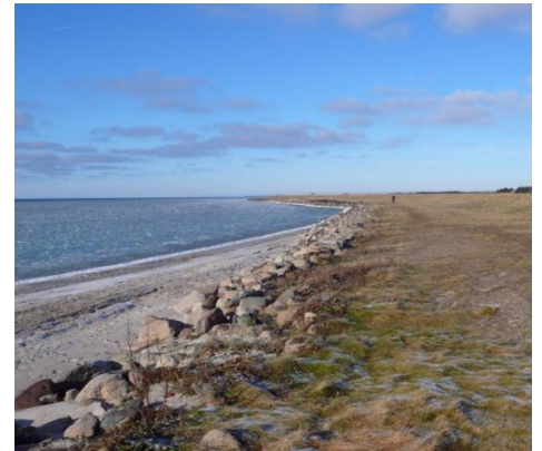
Figure 7.14 Revetment off the eastern end of Lalandia. Left: west end of revetment, remains of wooden pile groynes. Right: east end of revetment, sand accumulation west of Rødbyhavn has started
