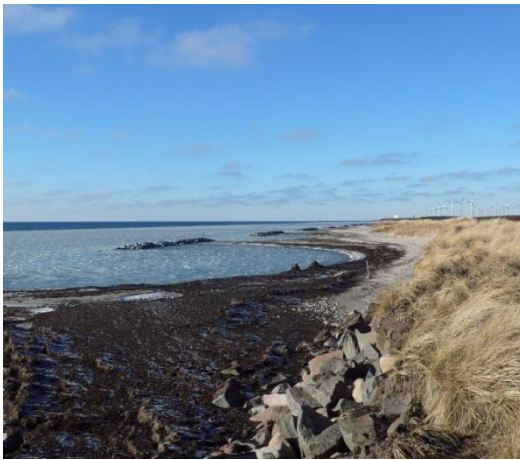
Figure 7.20 Breakwater scheme at Hyltofte Østersøbad. Upper left: west end of scheme. Upper right: pocket beach and tombolo within the scheme. Lower left: accumulation of seaweed in the eastern end of the scheme. Lower right: revetment and no beach SE of the scheme
