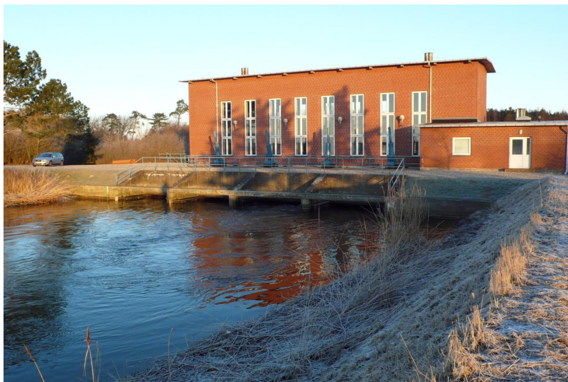
Figure 7.6 The "new" pumping station at Kramnitze built in 1966
