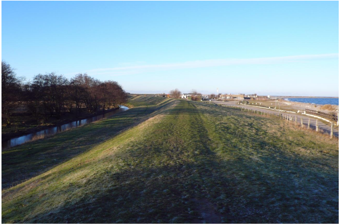
Figure 8.5 Dike at the east end of the westernmost of the three Binnensee lakes
