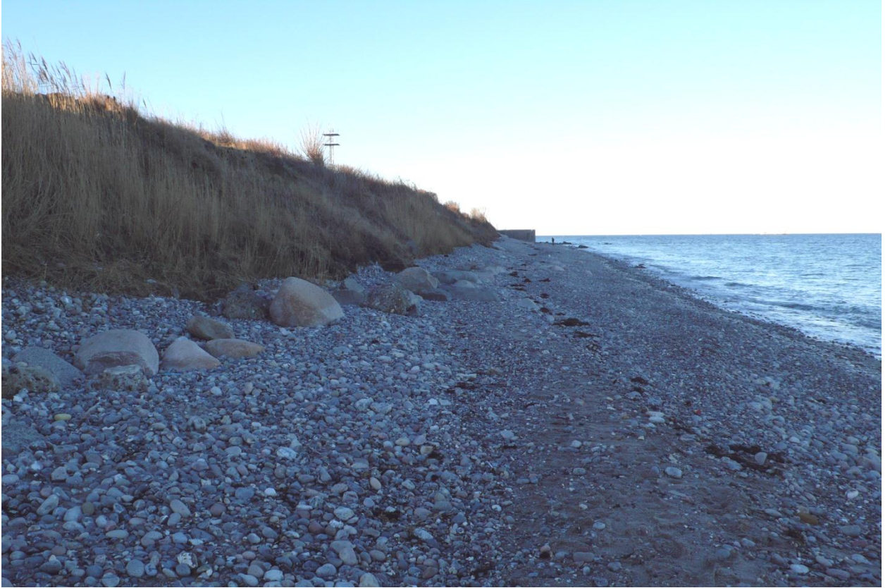
Figure 8.22 Cliff off Marienleuchte village, seawall at naval coastal station seen in the background. Shingle beach and a low revetment
