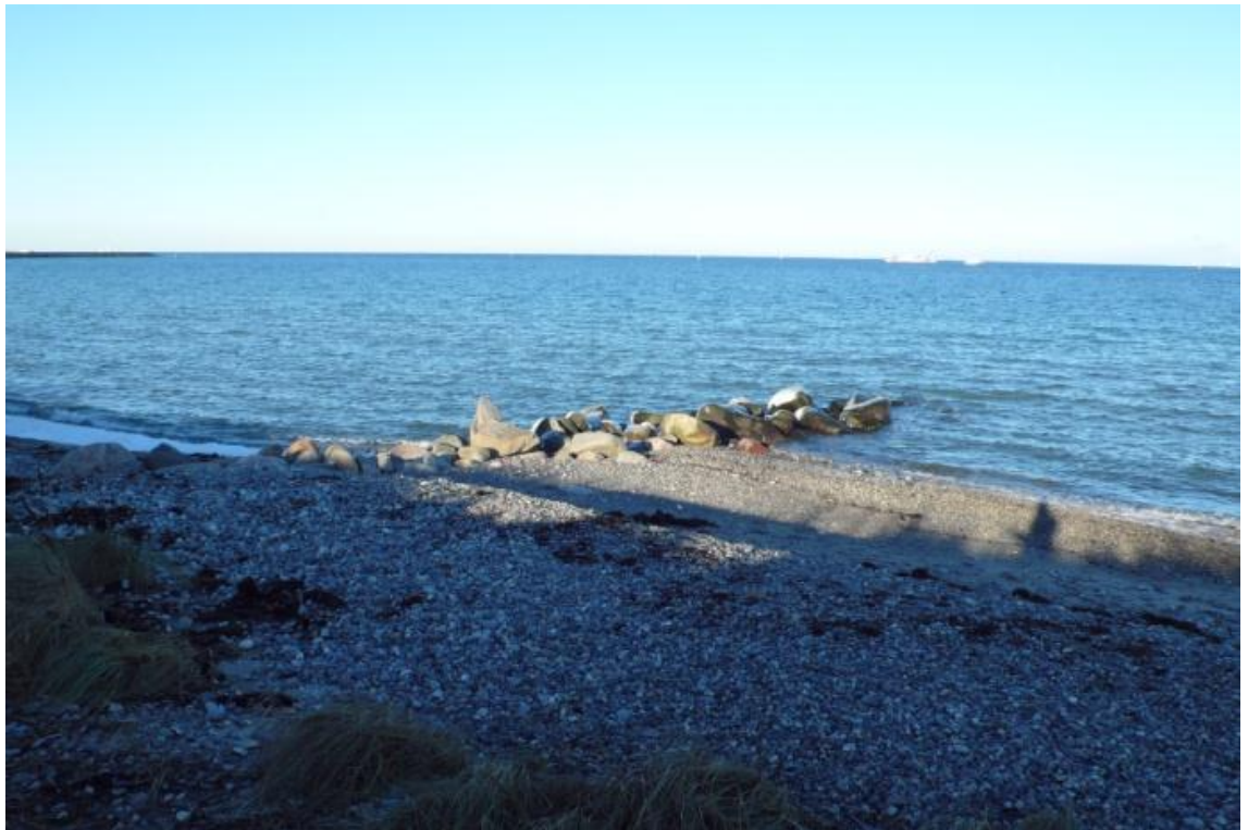
Figure 8.20 Stretch between Puttgarden and Marienleuchte. Shingle accumulation at groyne located NW of Marineleuchte
