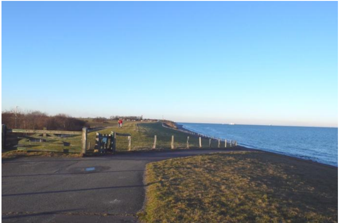
Figure 1.16 Dike between Marienleuchte and the till cliff off Klausdorf, protecting the low-lying land around Presen
