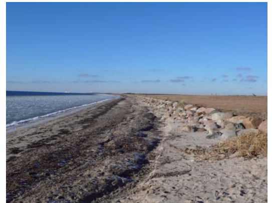
Figure 7.21 Stretch Hyldtofte Østersøbad to Brunddragene. Upper left: east end, breakwater scheme seen in the distant. Upper right: revetment in eastern end, remains of piled groynes. Lower left: middle part, sand undulation and buried revetment. Lower right: termination of revetment in east end of section, sandy beach takes over
