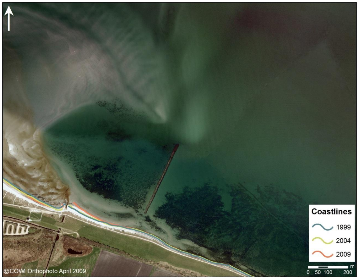
Figure 8.34 Recent shoreline evolution at the drainage outlet structure between Grüner Brink and the long detached groyne. Shorelines 1999, 2004 and 2009. Based on analysis of aerial photos, see Section 4.3. Aerial photo from 2009 (©COWI Orthophoto April 2009)
