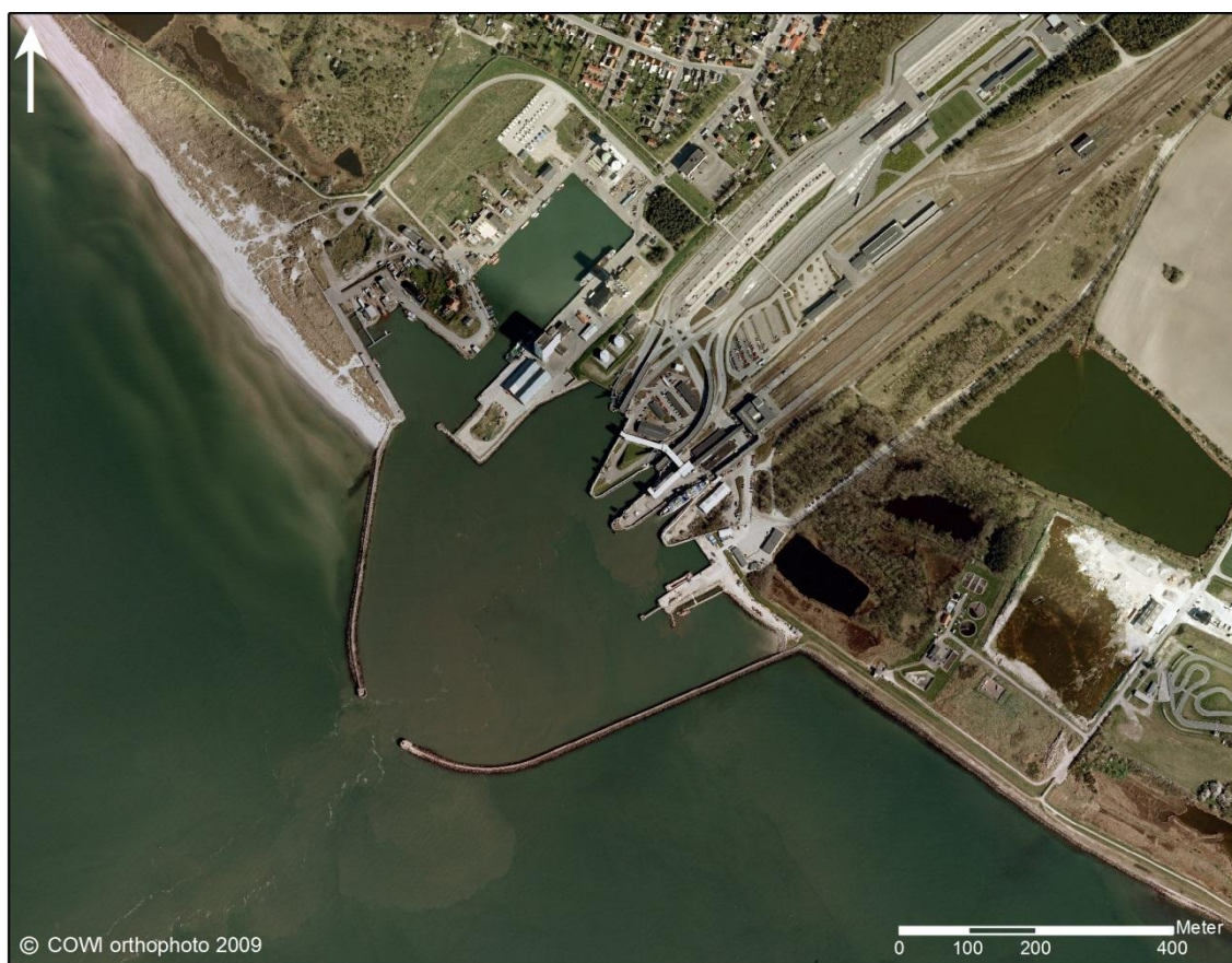
Figure 7.15 Rødbyhavn, consisting of the ferry harbour basin and some minor basins to the north of the ferry basin (the west basin and the north basin). Aerial photo from 2009 (©COWI Orthophoto April 2009)
