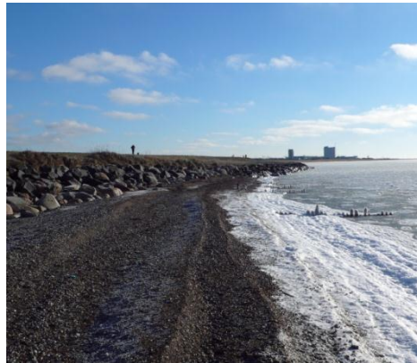
Figure 7.14 Revetment off the eastern end of Lalandia. Left: west end of revetment, remains of wooden pile groynes. Right: east end of revetment, sand accumulation west of Rødbyhavn has started
