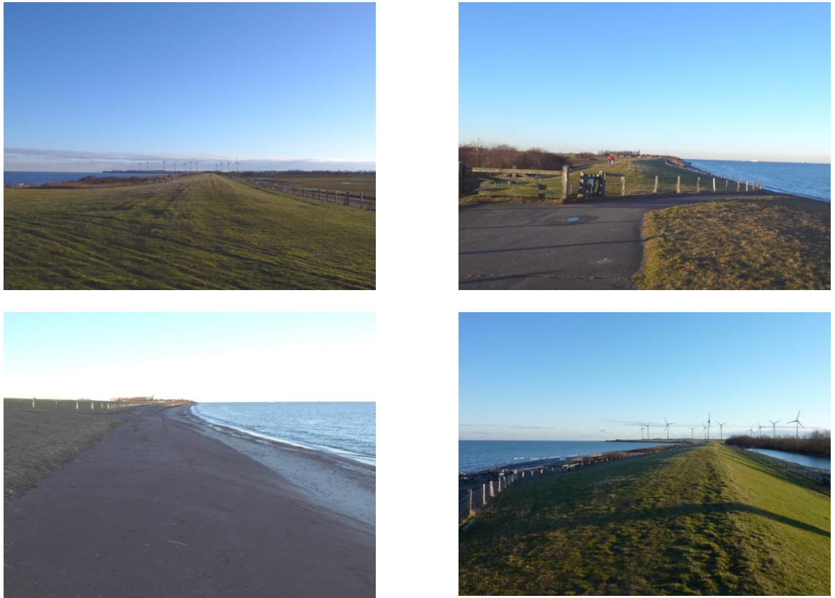
Figure 8.23 Dike between Marienleuchte and the till cliff off Klausdorf, protecting the low lying land around Presen. Upper left: northern end of dike immediately south of Marienleuchte. Upper right: southern part of dike north of pumping station off Presen. Lower left: asphalt revetment of dike north of drainage outlet at Presen, sandy/shingle beach off the dike. Lower right: dike from pumping station towards SSE, drainage canal along dike
