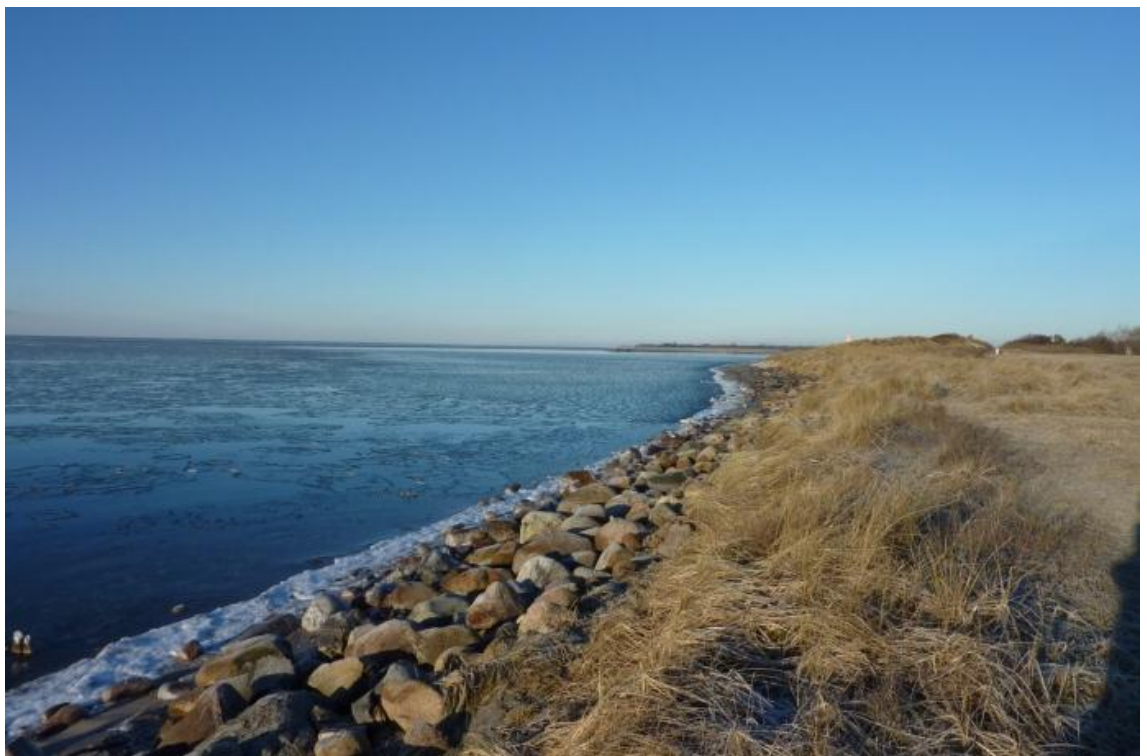
Figure 7.8 Revetment and no beach off the eastern part of Kramnitze
