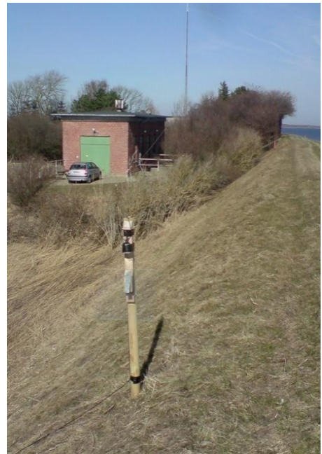
Figure 3-15 External microphone system at "Hyllekrog".
