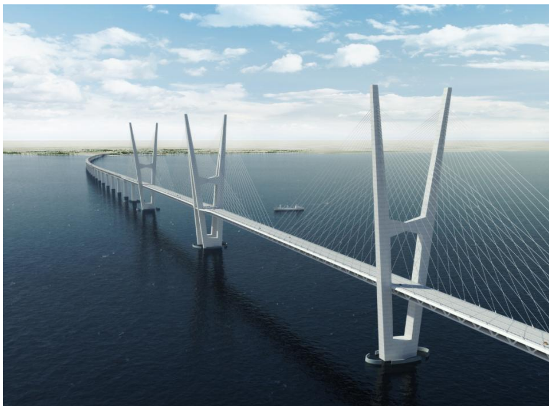
Fig. 2.8 Main bridge part of the cable stayed bridge
